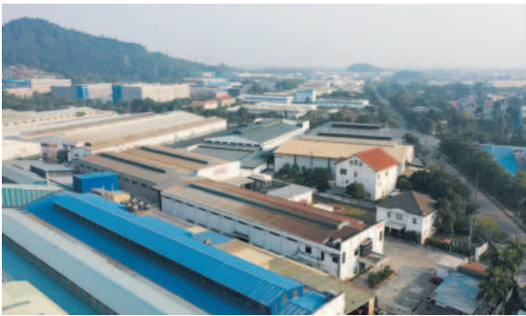
Khai Quang Industrial Park
