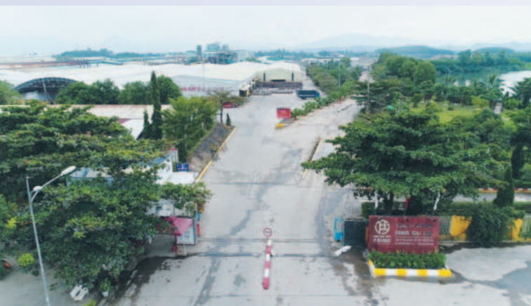
Overview of Prime Dai Loc's facility
