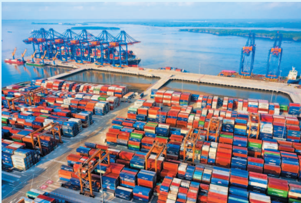
Binh Duong port, situated in the Southern key economic zone
